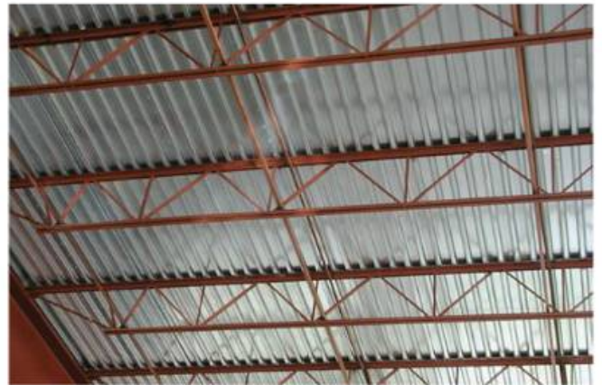
Figure 32 Bar joists.
