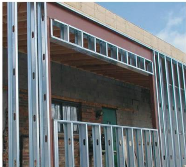
Figure 10 Steel stud wall section.
