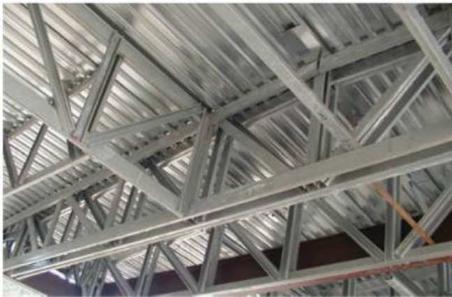
Figure 31 Metal roof trusses.
