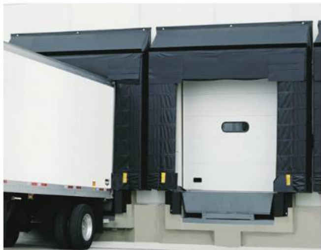
Figure 36 Thermally efficient door on a loading dock.
