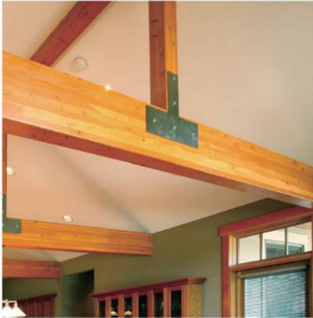
Figure 11 Glulam beam application.
