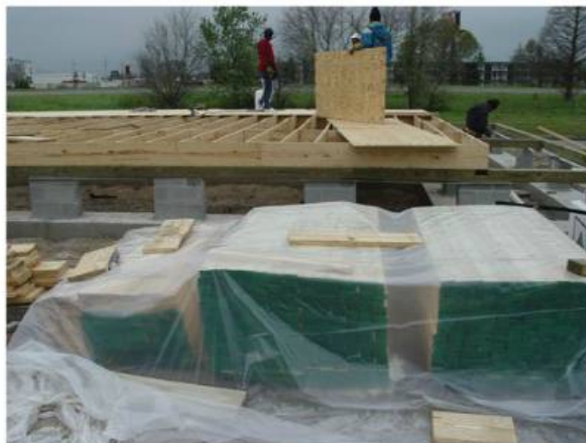
Figure 18 Storing plywood panels.
