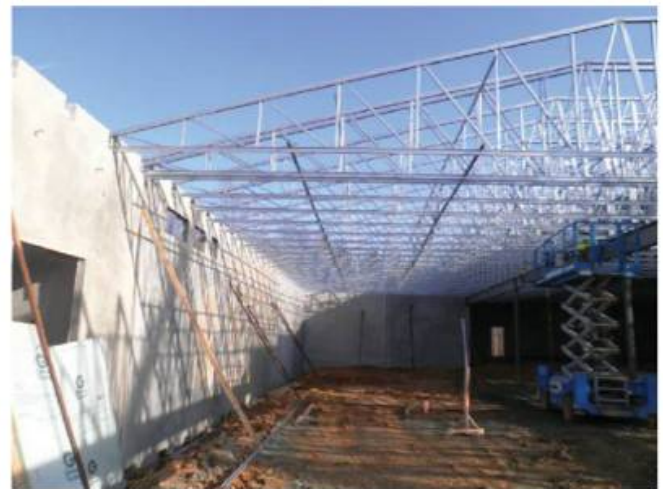
Figure 13 Steel trusses.
