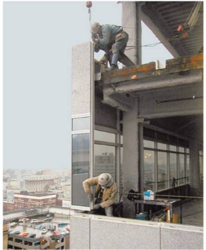
Figure 29 Installing a corner curtain wall panel.
