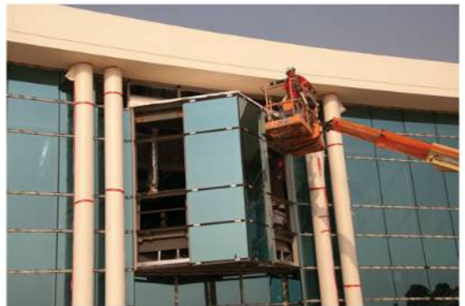
Figure 30 Curtain wall under construction.
