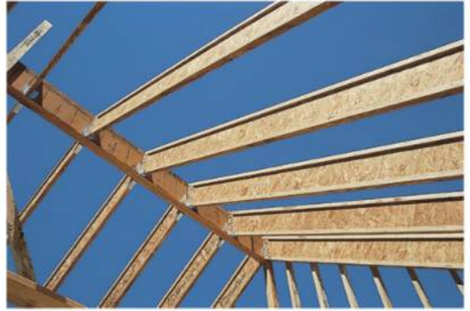
Figure 9 Wood I-beams.
